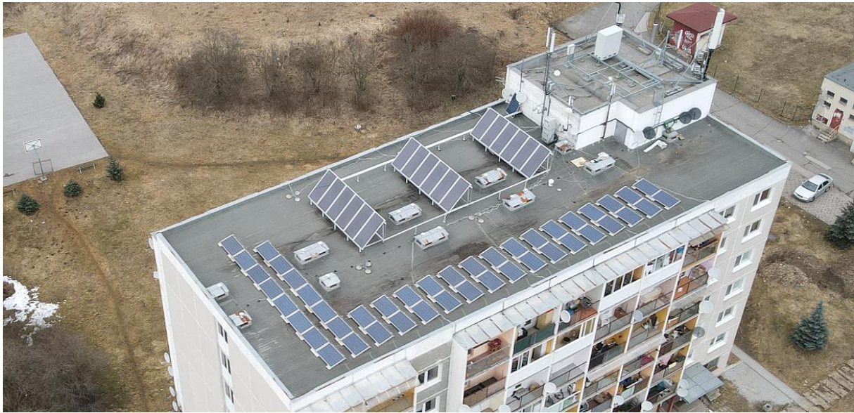
Figure 22 Solar and photovoltaic system on an apartment building in Spišská Nová Ves [30]
