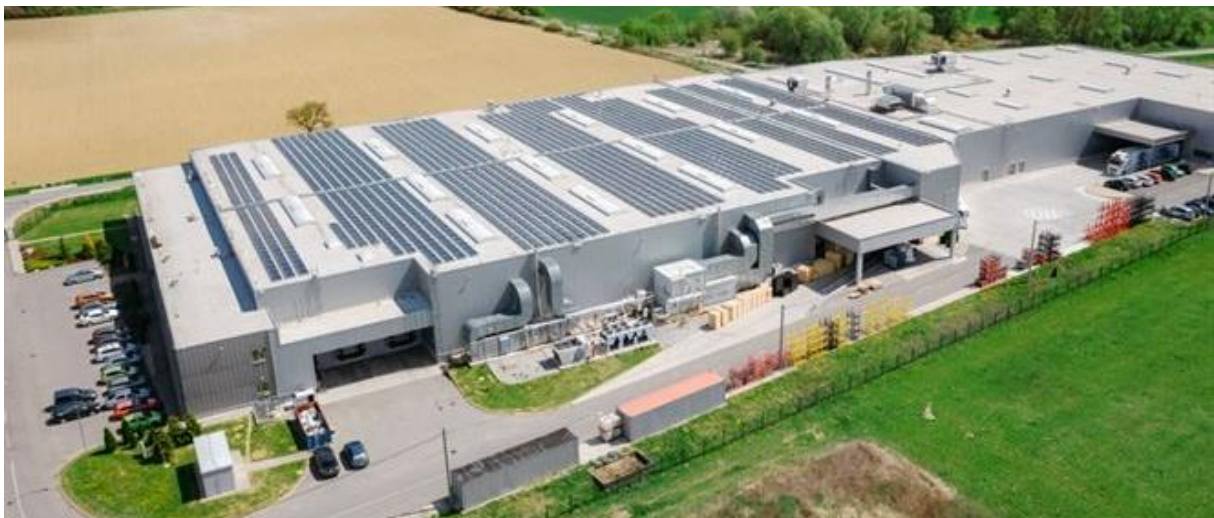
Figure 23 Photovoltaic system as a local resource in an industrial enterprise in Humenne [31]
