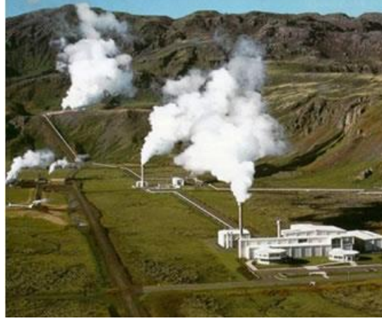
Figure 11. Kızıldere 3 Geothermal Power Plant
