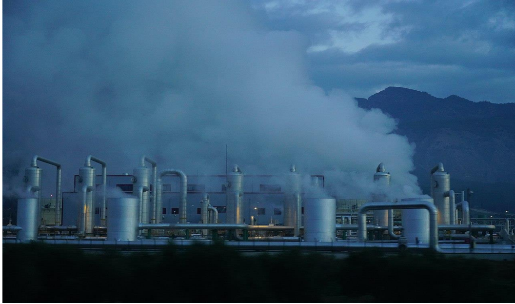
Figure 6. Kızıldere geothermal power plant in İzmir Province
